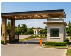
✓ Main Entrance Gate
